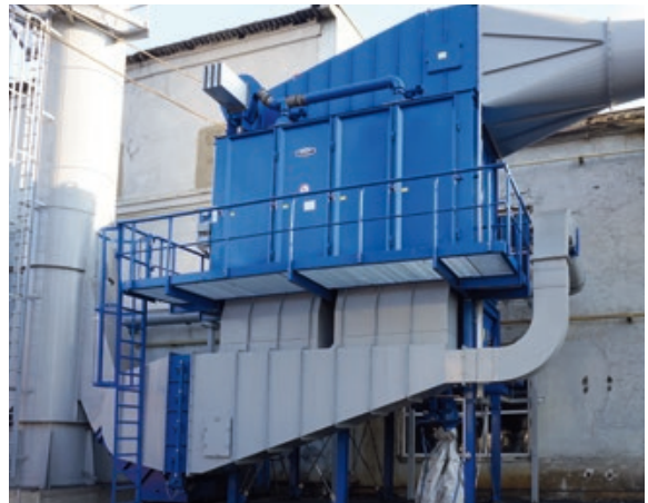
Entstaubungsfilter Dedusting filter plant
