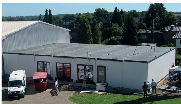
Erection of the new social amenities building
